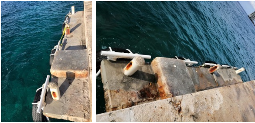
-Repaired Dock Surface by Ladder-
