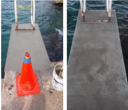
North Garage Gate Repair:
